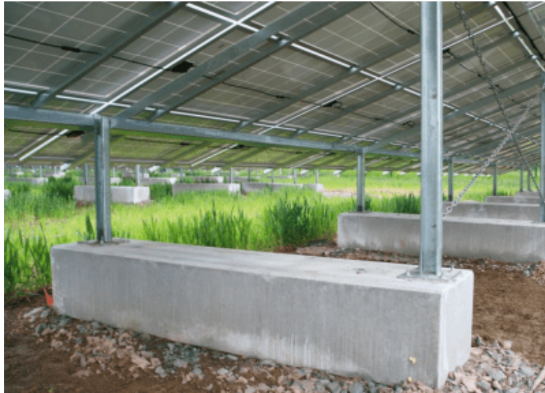
Figure 5-2: Typical Concrete Shoe Support
